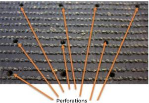
Artificial turf perforated for drainage
